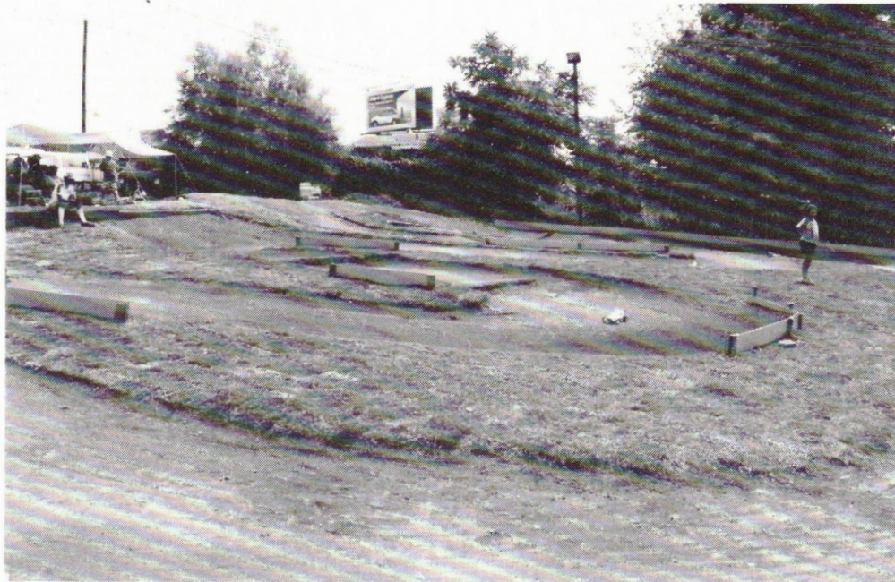
PDQ's national track. The track was made of red Georgia clay sprayed with calcium chloride to keep dust down and moisture in.
